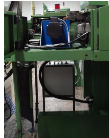
After the installation
